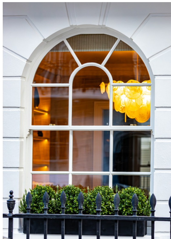
FIGURE A. TIMBER WINDOWS FROM PCW'S OWN JOINERY: AN ARCHED HEAD, SLIM GLAZING BARS AND SASH PROPORTIONS MATCHED TO THE HOUSE.
